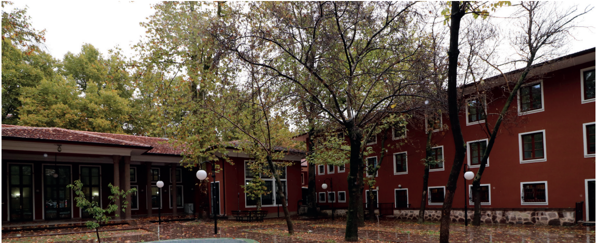
Figure 3. Building on Kumrular Street
