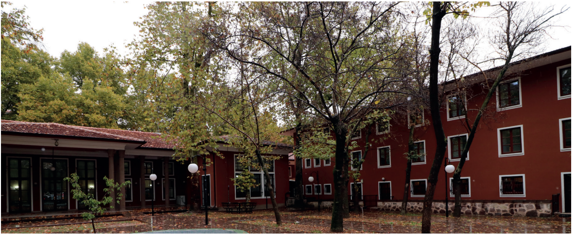
Figure 3. Previous Building on Kumrular Street (Adnan Ötüken Provincial Public Library)
