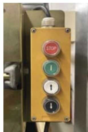
Goods lift in the stack room (Photo: Simon Lässer, FOBL)
