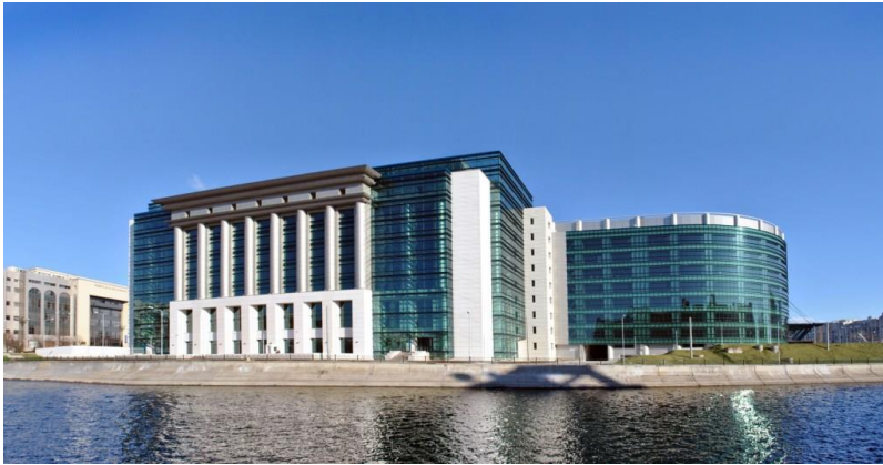
Exterior – the central headquarter
